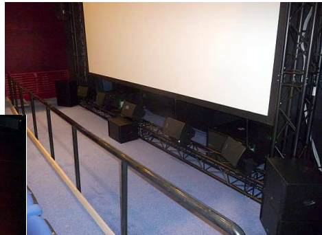
The SHV projector in place at the back of the cinema, and part of the 22.2 sound installation arranged around the projection screen
